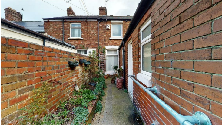
Rear yard with brick built storage.
